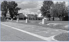
Concrete footings are the first step in erecting solar arrays at our schools.
